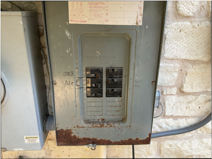
The main electrical panel box is not equipped with a main disconnect. Should have a main disconnect when six or more breakers are present.
