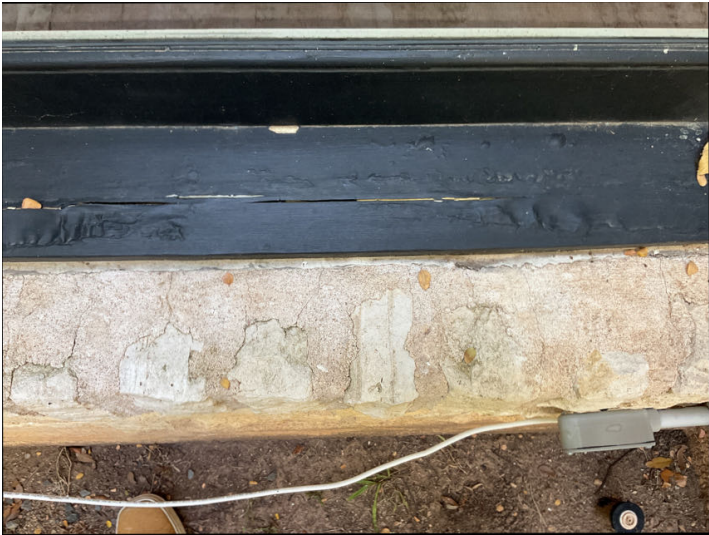
One or more wood sash window shows signs of water damage and or wood rot. Previous repairs.
