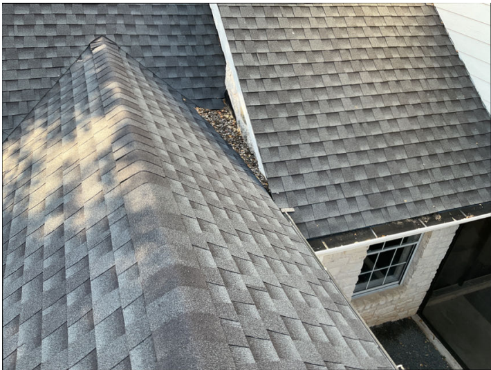
Debris on the roof surface observed in one or more locations.
