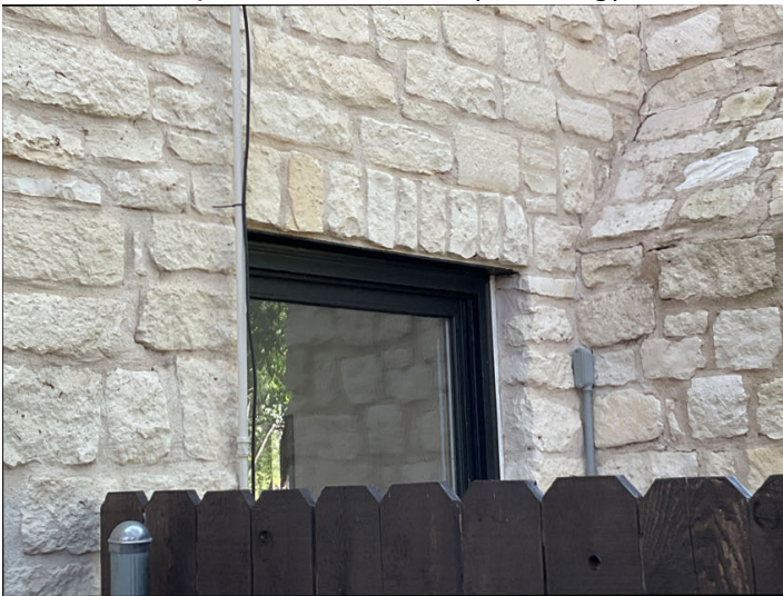
Lack of weep holes in rock mortar above windows. Common to see you on older homes.
