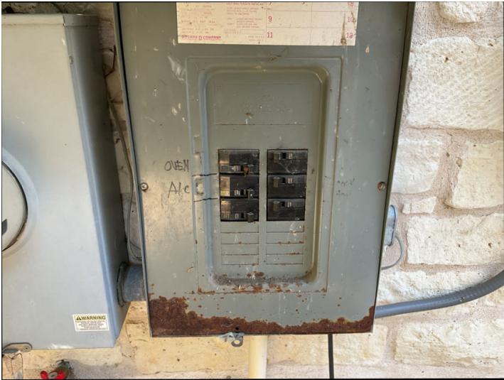
The electrical panel should have 30 inch clearance on both sides and 36 inch clearance in front of the electrical panel.
