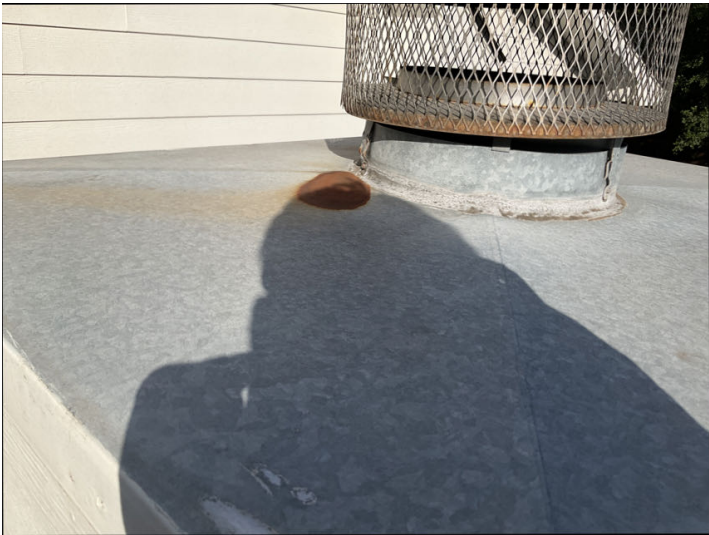
One one or more chimneys. Metal is rusty: The metal crown or cover at the top of the chimney is shows signs of excessive rust. Holes or pits in the metal may develop, which in turn may allow water into the chimney chase.
