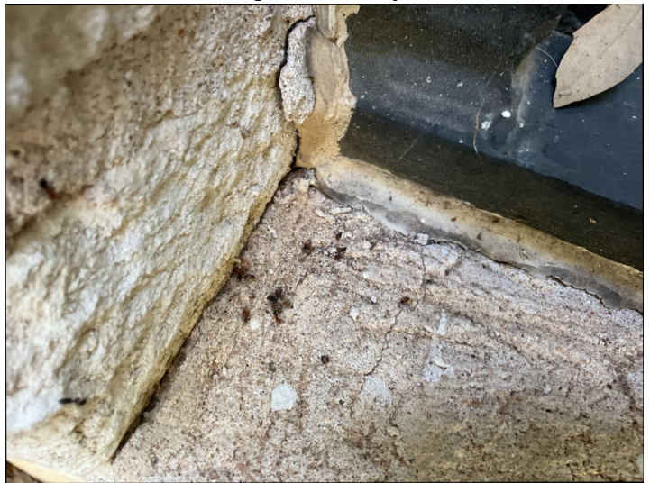
-Exterior window trim has missing or deteriorated sealants (caulking) where the window frame meets the wall cladding and or trim.
