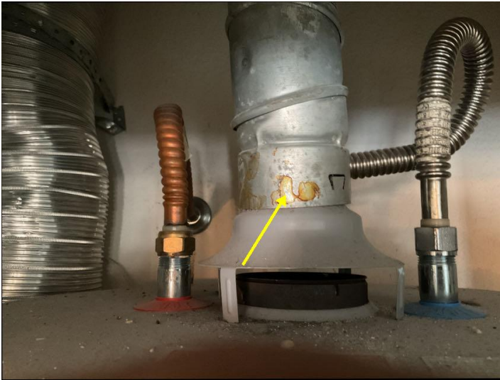
The water heater vent pipe is not screwed to the draft hood.
