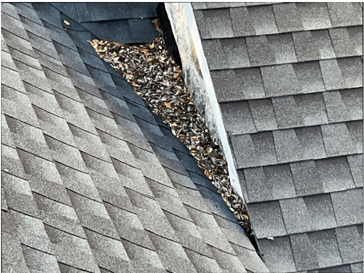
Poor flashing and or roof design observed on the right back corner. Debris lodged in valley flashing.
