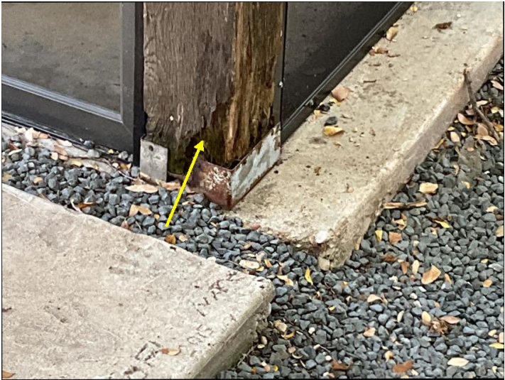
One or more back patio wood columns shows signs of water damage and wood rot at the bottom.
