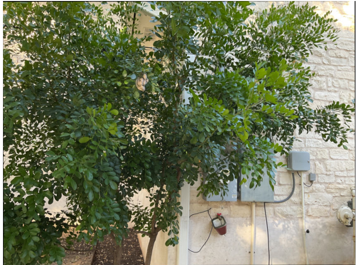
There is foliage in contact with the exterior walls. Foliage should be trimmed and maintained away from the house to prevent damage to the exterior wall coverings and to eliminate a condusive condition for wood destroying insects.
