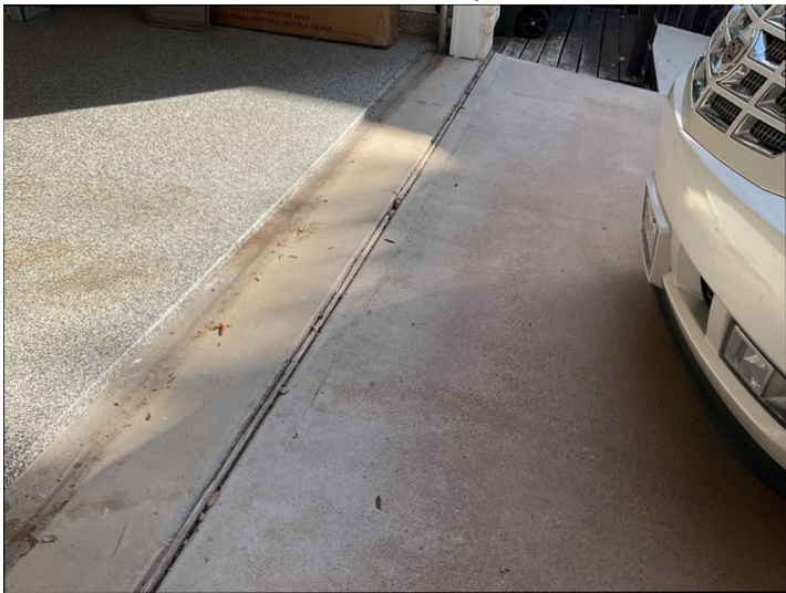
The driveway has settled at the garage opening.
