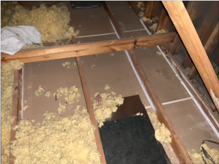
Attic insulation is missing in one or more locations. Attic insulation is missing in one or more locations.
