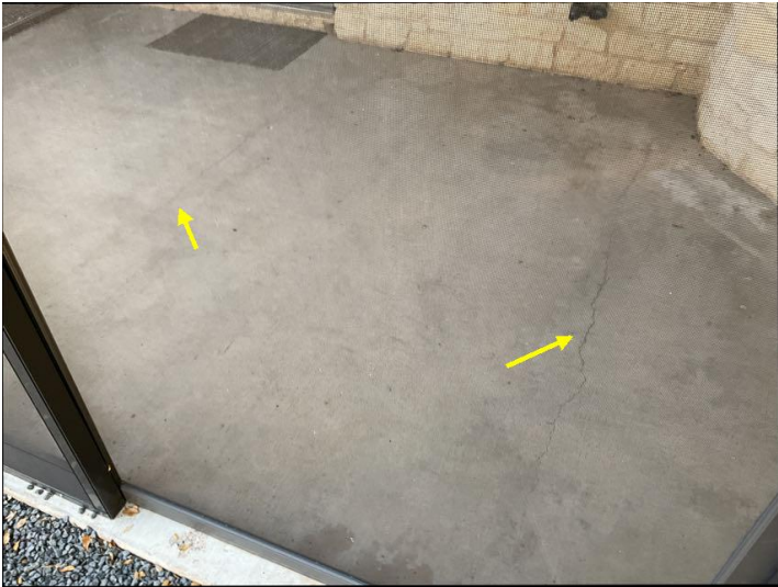
Cracks observed in back patio concrete services in one or more locations.
