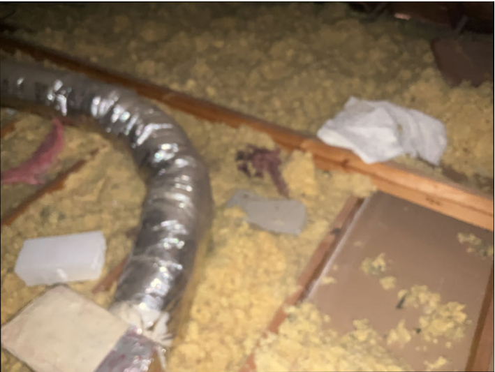
Attic insulation is missing in one or more locations. Attic insulation is missing in one or more locations.
