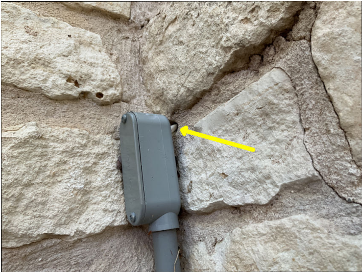
Exterior wall penetrations have missing and or separated sealants (caulking).
