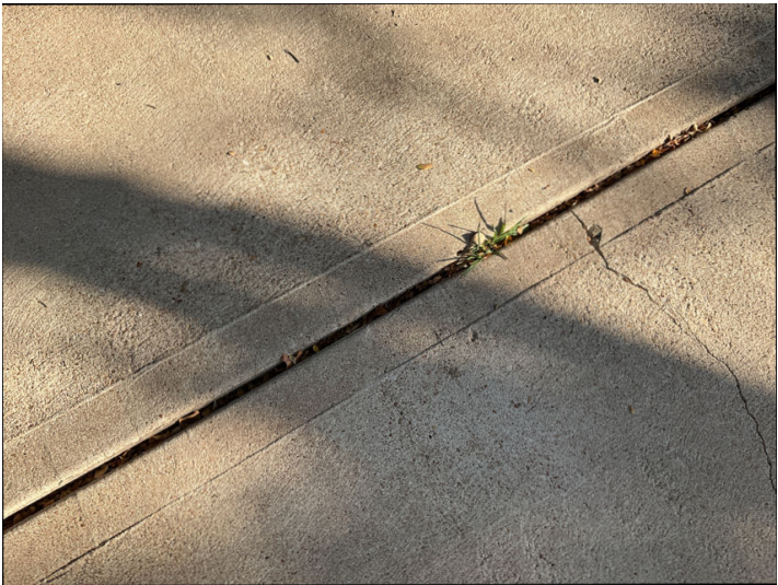
Driveway concrete expansion joint wood material is missing and or separated in one or more locations.
