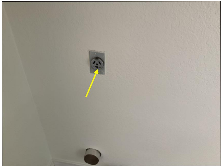
Clothes dryer electrical receptacle is a 3 prong receptacle without a ground. Newer dryers use a 4 prong receptacle. May need to update the receptacle for your dryer.
