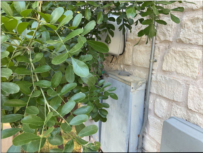
The electrical panel should have 30 inch clearance on both sides and 36 inch clearance in front of the electrical panel.
