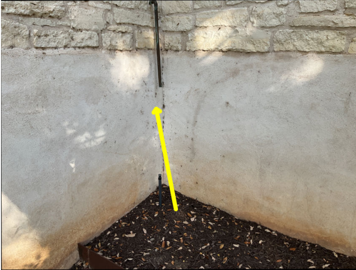
Water heater temperature and pressure drain line to terminate within 6 inches of the ground.
