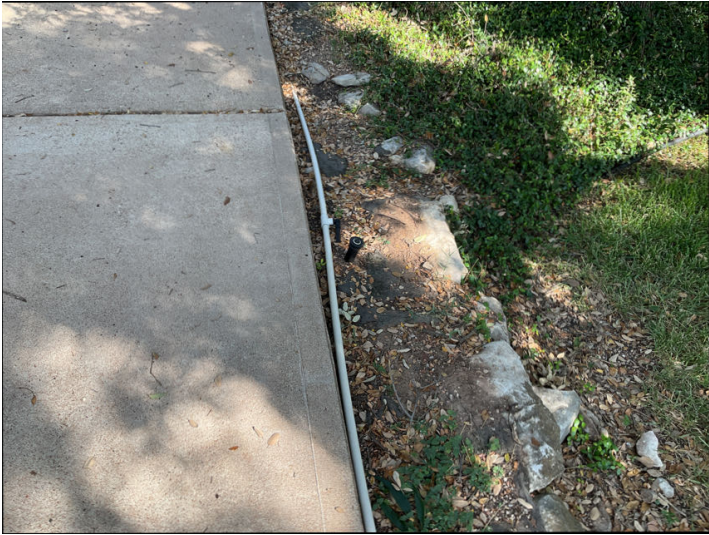
Exposed sprinkler lines observed on the right side of the driveway.
