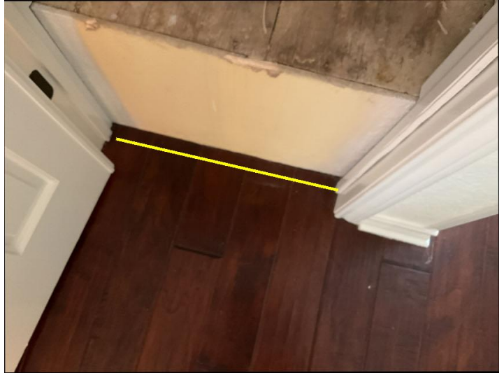
Door to Water heater closet should have a door seal at the bottom. Water heater is utilizing living space air for combustion venting. Safety hazard
