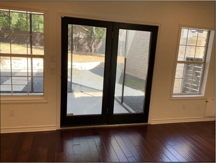
Windows on both sides of the back right door or not labeled as safety of tempered glass. Should be tempered glass When within 24 inches of the opening of the door
