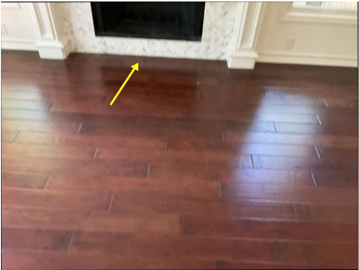
The front left a formal living room fireplace is not equipped with a fireproof heart in front of the opening.
