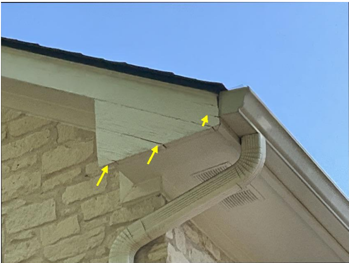
Wood fascia trim is checking and or splitting in one or more locations.
