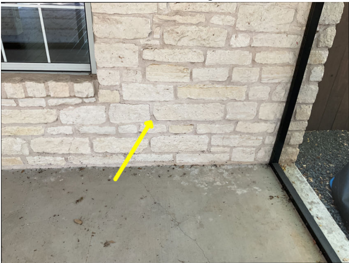
Stairstep crack in rock mortar on back patio right side.
