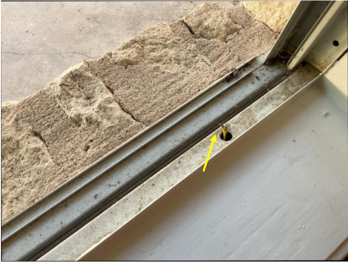
Window frames have been drilled on the exterior bottom on the frame for security sensors. Drill holes can allow water to enter into the wall envelope. Hole for sensors should be properly sealed to prevent water and or moisture from entering the wall envelope.
