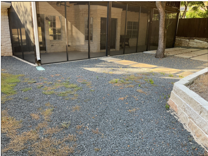
Negative grade or (poor soil grade) was observed, ground surface slopes towards the foundation or has less than 2% grade away from foundation. To keep surface water from collecting up against and or near the foundation grading should have a 2% slope (6 inches within the first 10 feet) away from the structure.
