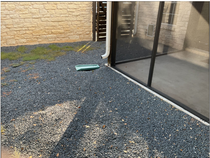
One or more gutter downspouts do not terminate all the way to the ground. Raised too high.
