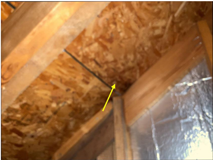
Water stains observed on roof decking in one or more locations.
