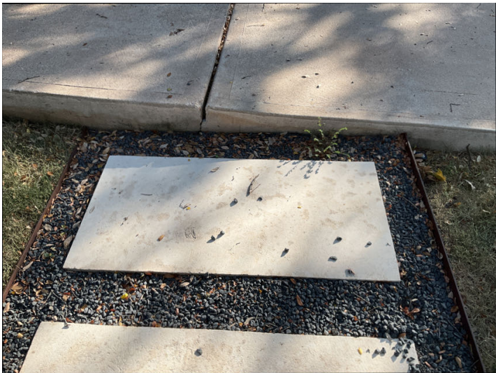
Front sidewalk concrete surface is below driveway surface Potential trip hazard.
