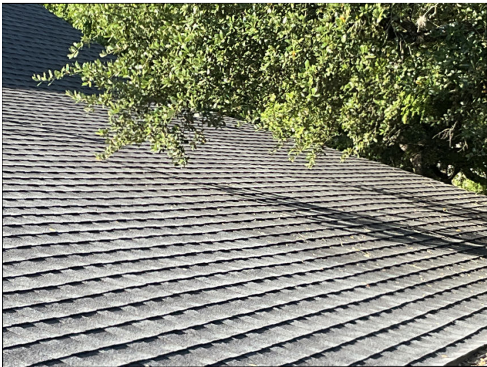
Trees should be trimmed away from the roof structure to prevent trees from rubbing the shingle surface and to help keep rodents and animals from accessing the roof structure.
