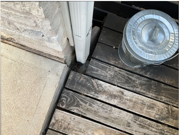
The attic space in the garage cannot be access due to owners belongings in the way at the time of the inspection. The gutter downspout is missing on the right side of the garage. Recommend installing splash block.
