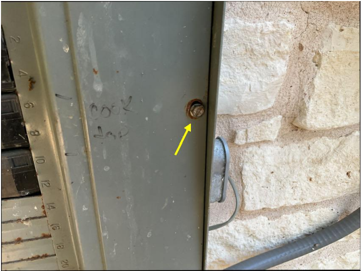
The panel box dead front cover screws should be blunt tipped. Safety hazard.
