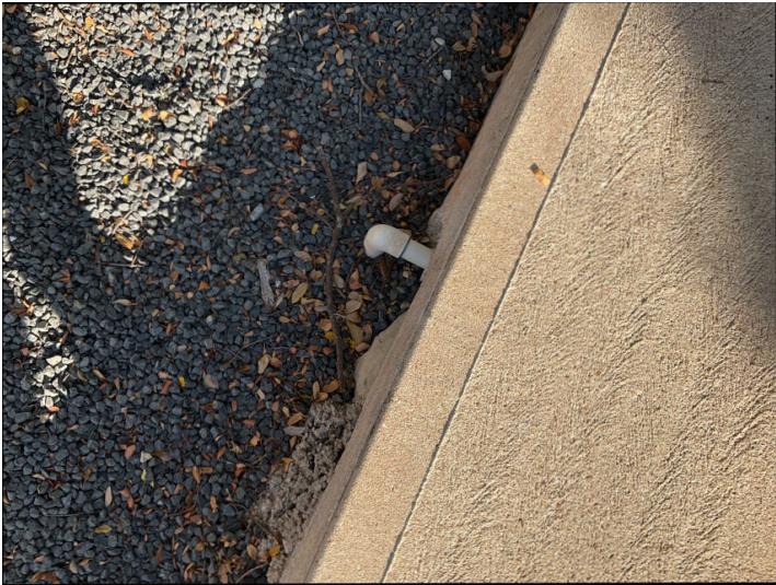
Exposed drip irrigation water lines observed in one or more locations.
