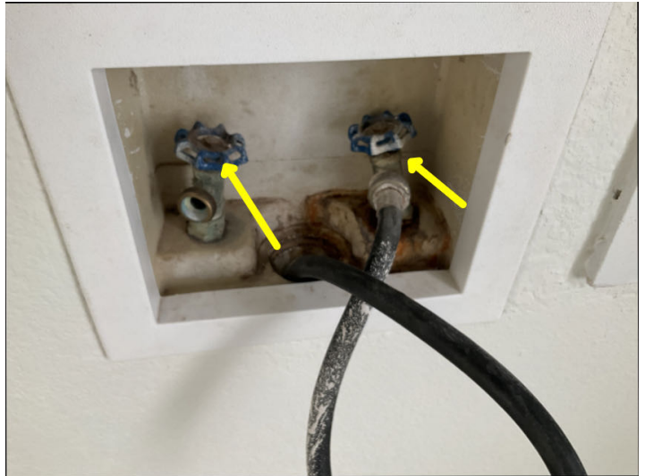
Washer supply hose bib Lineslook at the valve stems when I opened.
