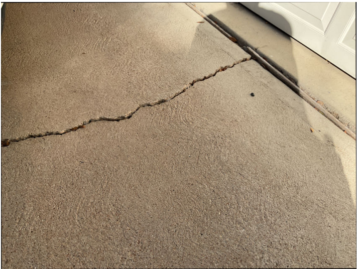
Cracks in driveway concrete surfaces in one or more locations.
