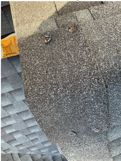
There are exposed fasteners on the roof. Sealant should be applied to exposed fastener heads to prevent moisture from penetrating the roof in those areas.
